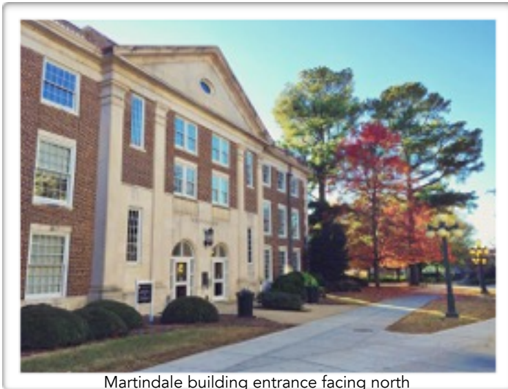
Martindale building entrance facing north
